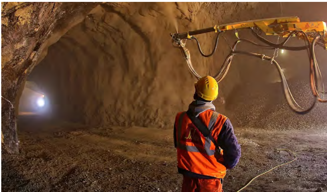
Figure 60: Sprayed concrete (shotcrete) installation in an underground mine ( www.sika.com/en/solutions-for-projects/mining.html )
