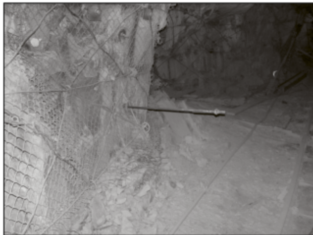
Figure 37 Cable Lacing in a South African Mine (Hadjigeorgiou & Potvin, 2011, p. 579)
