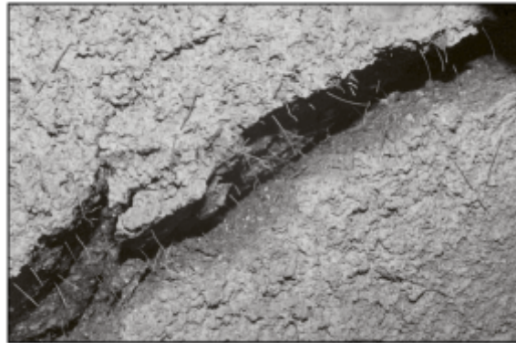
Figure 38 Fibre-reinforced Shotcrete, Showing Fibres Bridging Cracks (Hadjigeorgiou & Potvin, 2011, p. 581)
