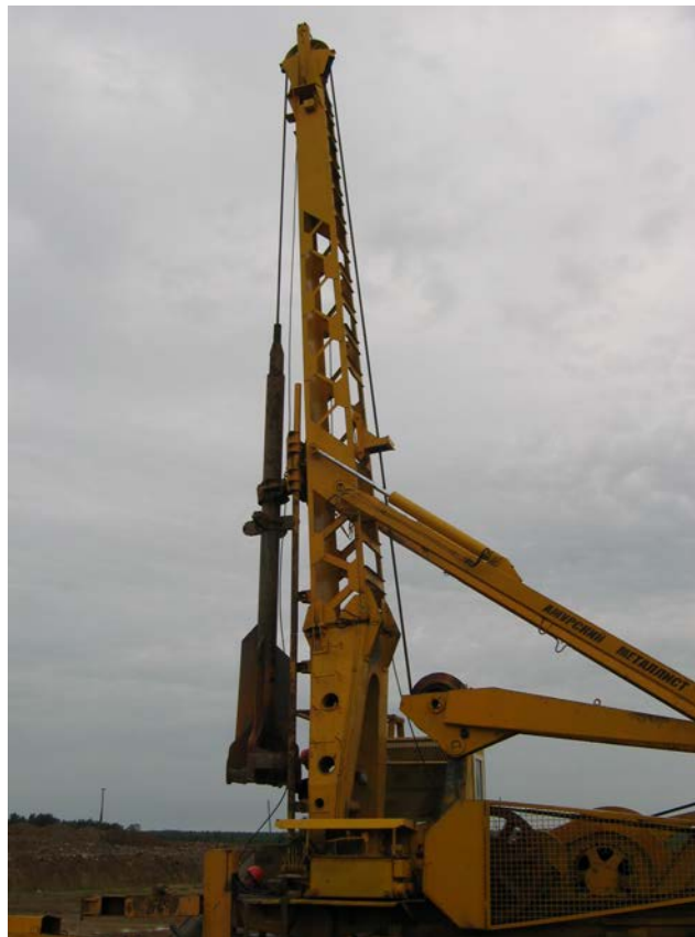
Figure 5.1: Rig for drilling 1-metre diameter holes.
